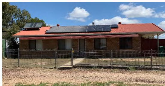
Figure 5.6: Brick veneer on concrete slab on ground and metal roof
