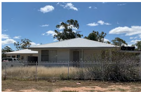
Figure 5.5: Timber framing on concrete slab on ground and metal roof
