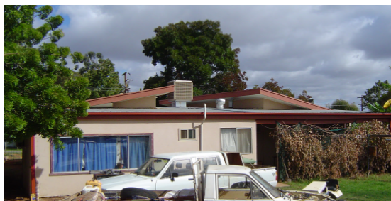
Figure 6.4: Brick veneer on concrete slab with metal roof, Dareton
