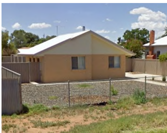
Figure 6.4: Brick veneer on concrete slab with metal roof, Dareton
