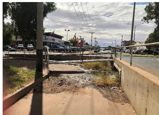
Figure 3.12: Typical stormwater culvert
